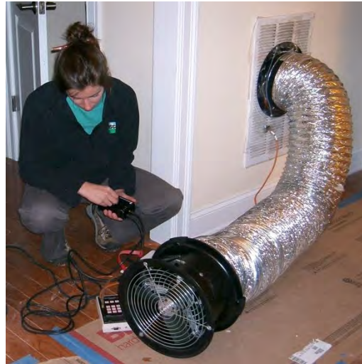
Duct Leakage Test
